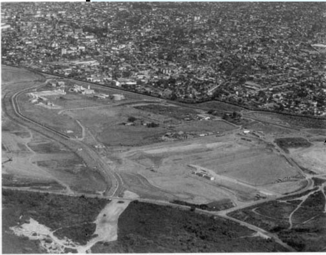
Standing alone just north of the burgeoning metropolis of Tijuana, the International Treatment Plant can be seen just completed in the center, left of the photo. The City of Tijuana has experienced phenomenal growth since its awaking from the small, sleepy town of 1941. (see photo page 36) (Courtesy City of San Diego)
