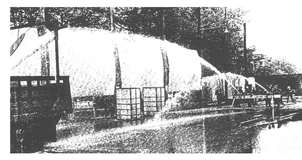
"... the increase in water flow by adding only 30 wppm of Polyethylene oxide (PEO) allows firemen to deliver the same amount of water to a higher elevation from a 1.5-inch hose which can be handled by two men, instead of four men to handle 2.5-inch hose fed only by water ..."
