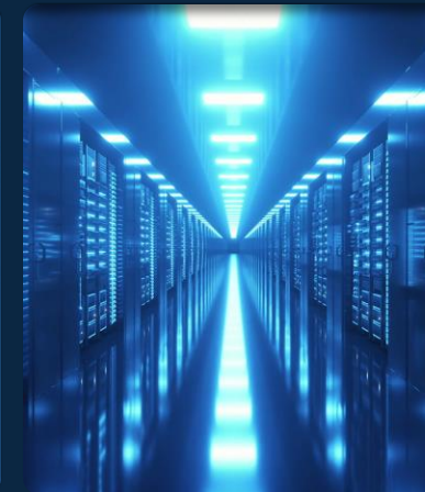
Wireless data center
