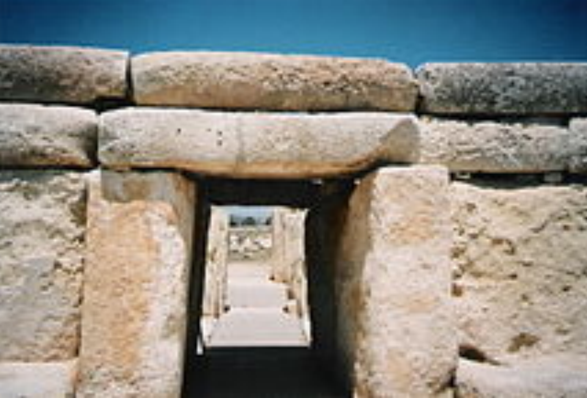
The entrance to a temple in Malta: Large stones are needed to support the top of the gate
